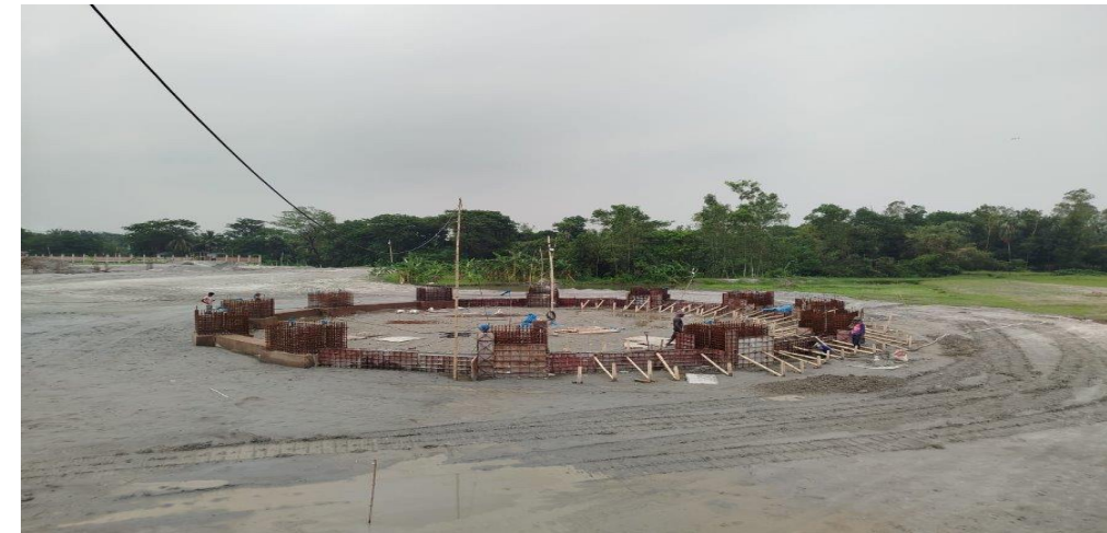
Dhaka Plant Construction
